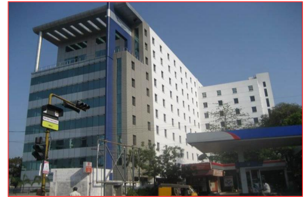
Fortis Hospital, Chennai
